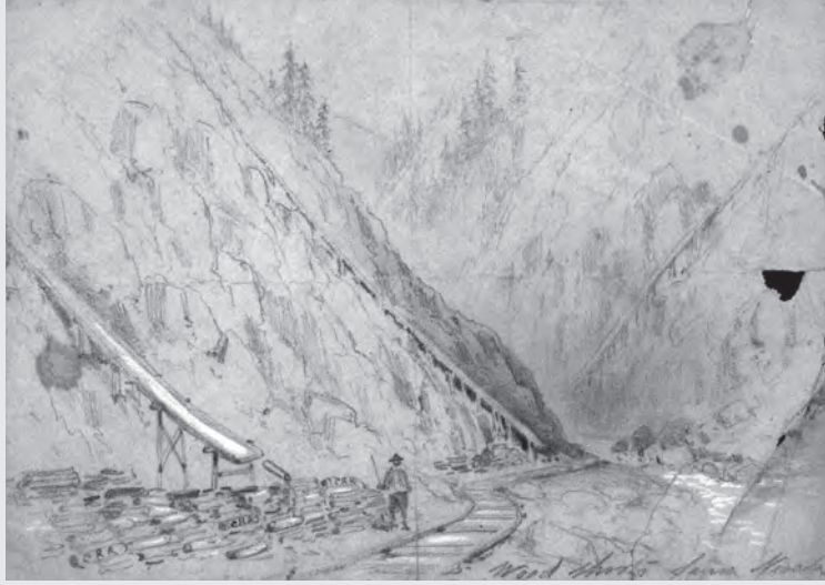
3.7 Wood chutes, Central Pacific Railroad, Sierra Nevada.
