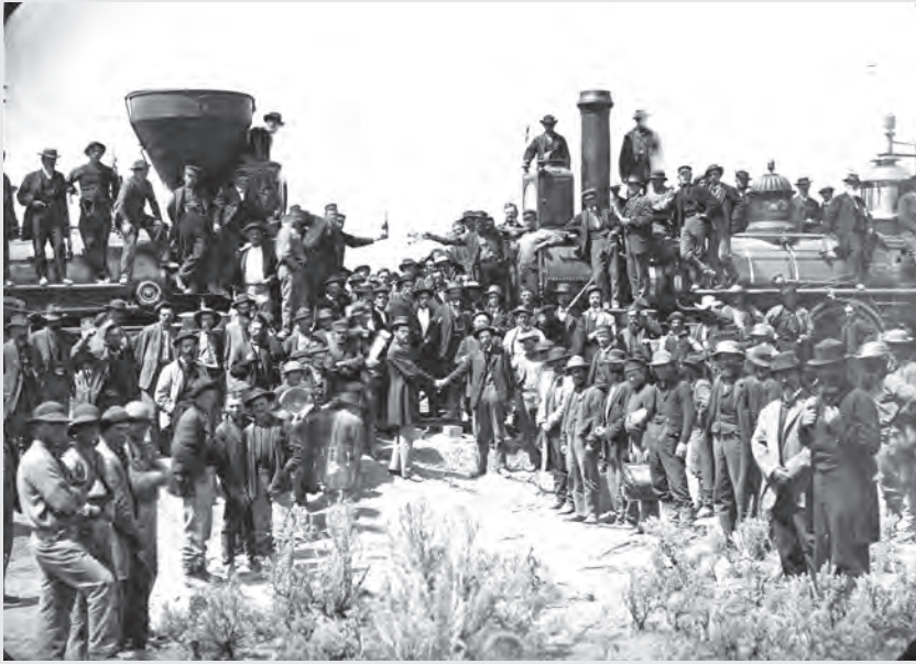
3.1 Joining of the rails, Promontory Summit, Utah, May 10, 1869. Note the different smokestack designs of the Jupiter (left) and No. 119 (right) an indication of the wood-to-coal energy transition under way.
