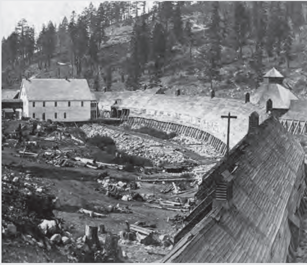
3.5 Central Pacific Railroad snow sheds at Summit Station in the Sierra Nevada. Note the forests, stumps, logs, wooden structures, and smoke vents.
